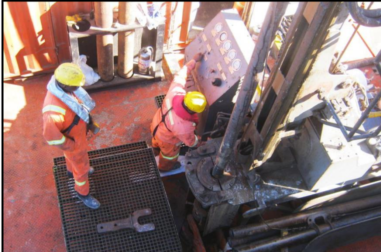
Drilling 25m hole takes max 2 hours
